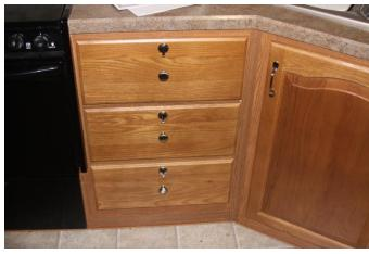
solution was to purchase the little stick on felt circles and attached them to the corners of the drawer which took up the space resulting in a tight fitting drawer.
