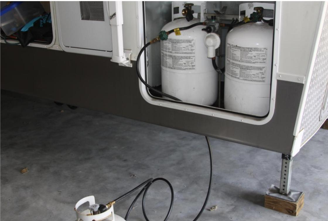
And this is of the male Acme fitting screwed into the regulator pigtail providing gas to run the generator.
